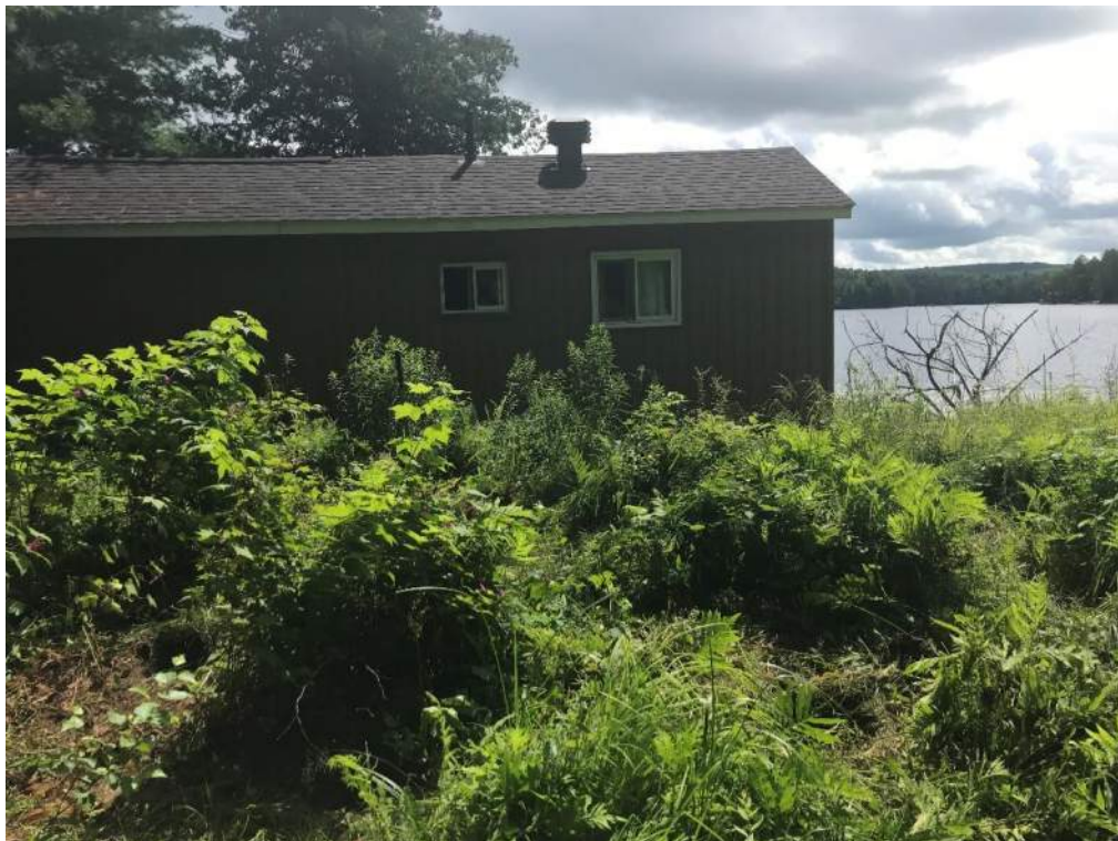
Photo 2 – Proposed area of development and existing bunkie (July 7, 2023).
