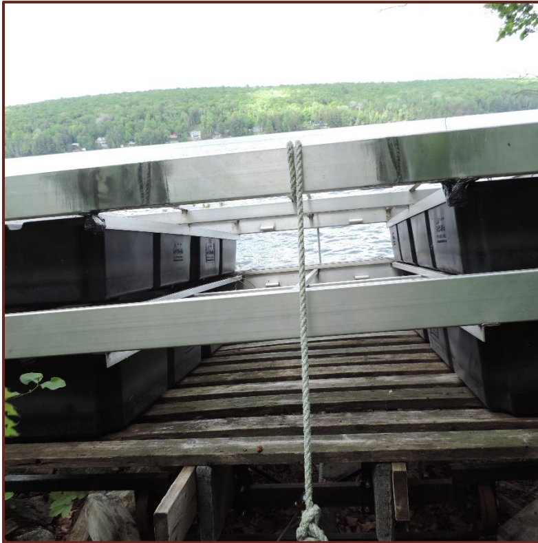
Photo 9. View of the boat rail located close to the water.
