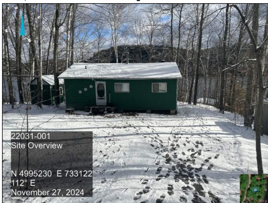
Photo 2 Site overview, looking east, showing a residential building and small building at the top of the slope and mixed mature trees.
