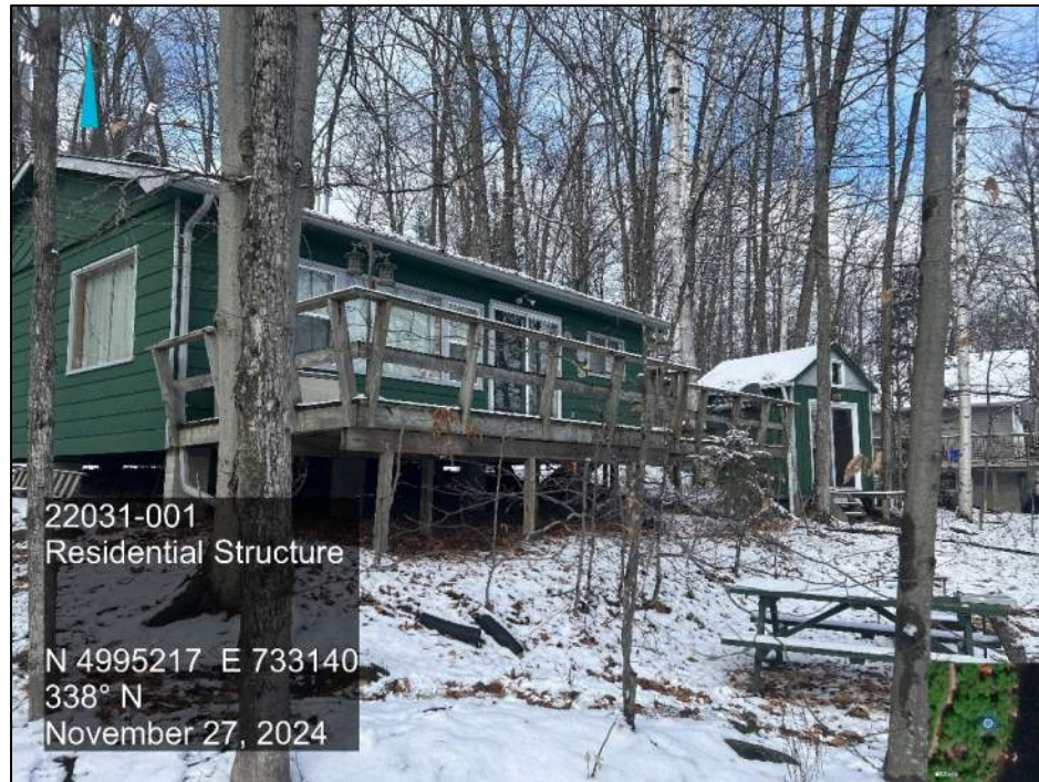
Photo 3 Site overview, looking northwest, showing a residential building and small building at the top of the slope and mixed mature trees.
