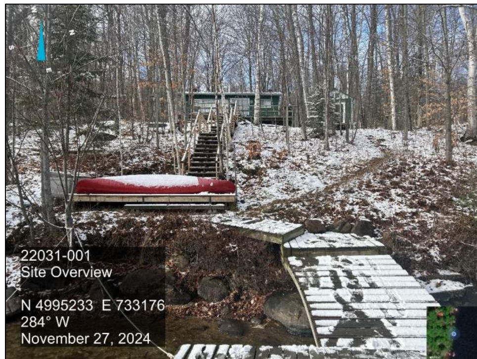
Photo 4 Site overview, looking west, from the dock, showing a residential building at the top of slope, staircase along the slope, dock along the base of slope, and mixed mature trees across the site.
