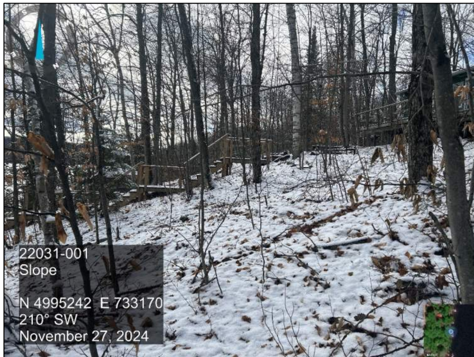
Photo 8 View of the slope face, looking south, showing mixed mature trees, staircase, and a residential structure.
