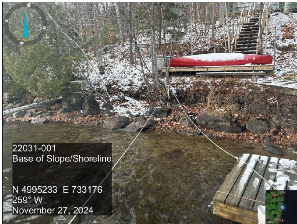
Photo 11 View from the dock, looking west towards the base of the slope/shoreline, showing mixed mature trees, a dock, and a staircase. Large boulders exposed along the base of the slope.
