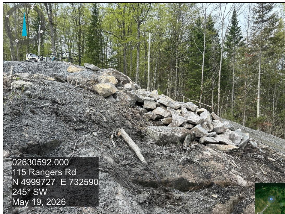
Photo 4 View of top of the bedrock slope, looking west, showing granite and stockpiled boulders along the top of the slope.
