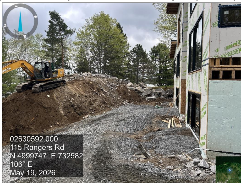
Photo 8 View of bottom of the slope, north of the residential structure under construction, looking east. Showing mixed mature trees along the shoreline and gravel over top of the bedrock. A large stockpile of construction debris and boulders is evident above the shoreline.
