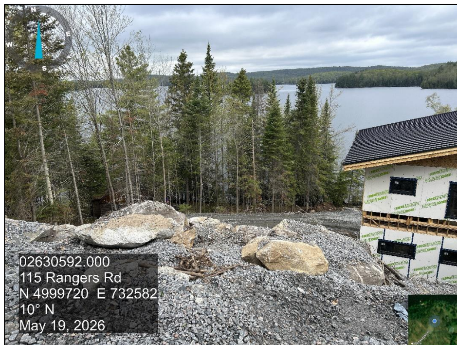
Photo 10 Site overview, from the top of the slope looking north towards Baptiste Lake. Showing the residential structure under construction and boulders along the top of the slope.
