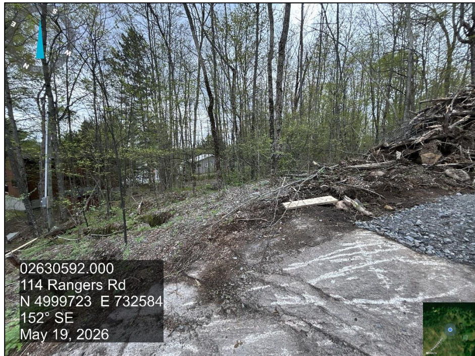
Photo 3 View of top of the bedrock slope, looking east, showing granite and stockpiled construction debris and trees.
