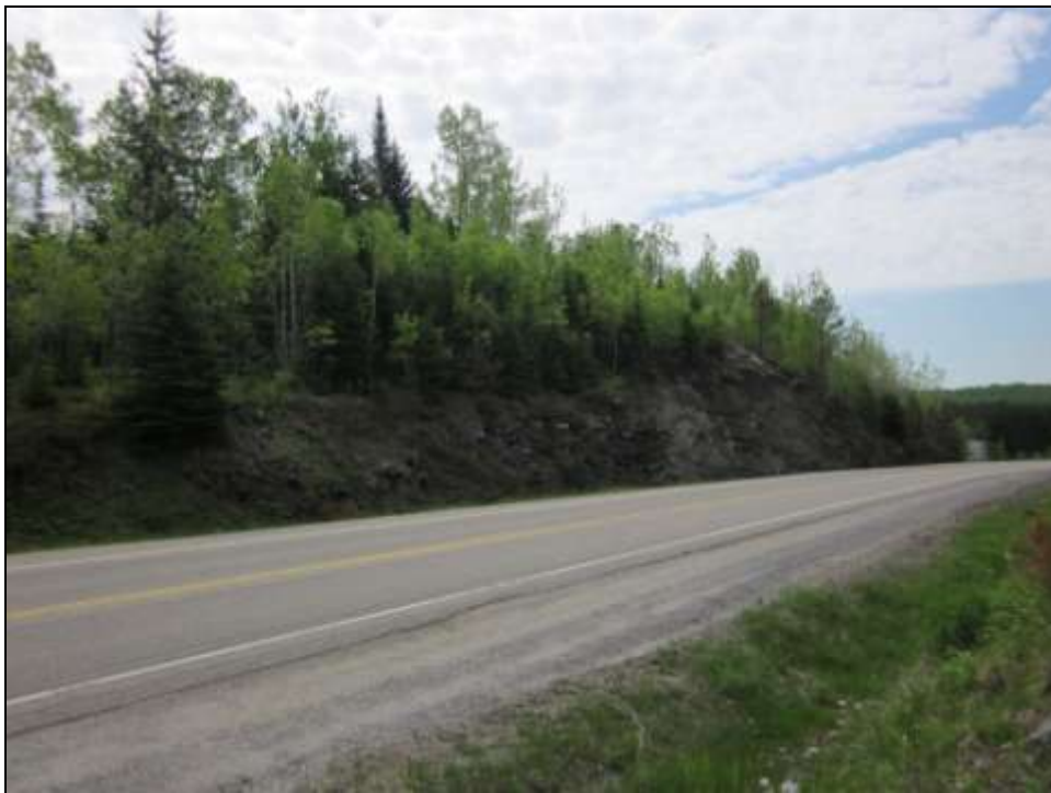
Image 5.4: Oriented SE, Elevated Area of Buck Hill Abutting Highway 62
