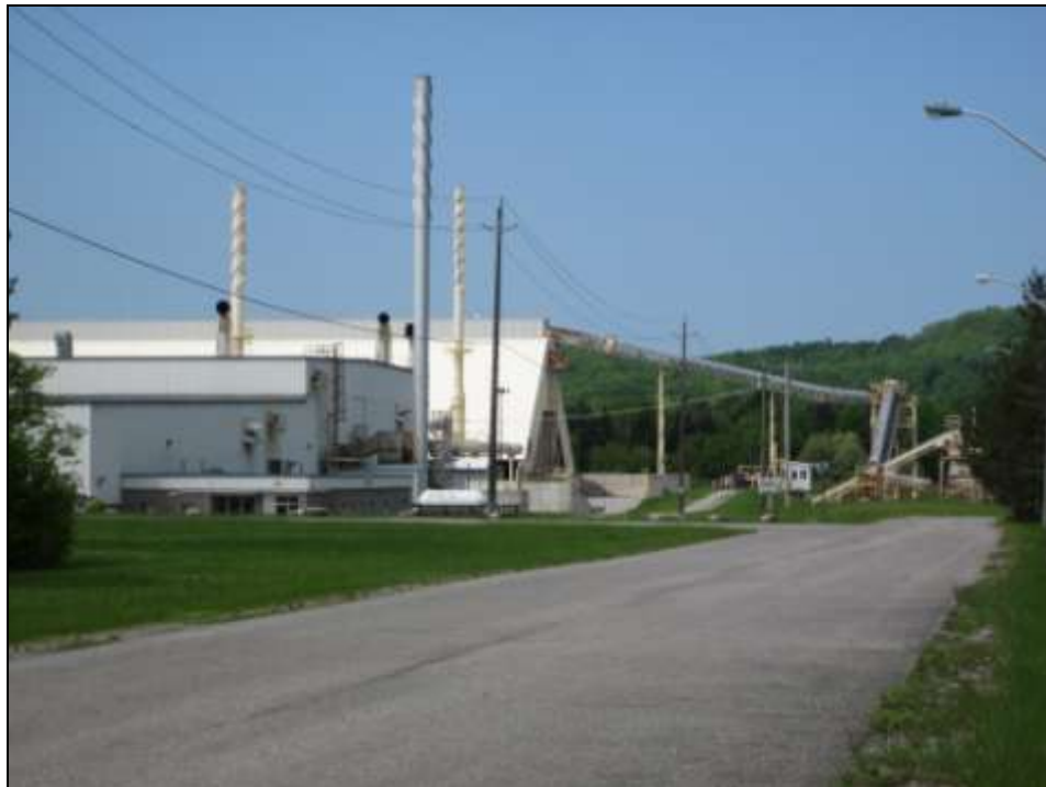
Image 5.8: Oriented W, Large Wood Product Processing Facility
